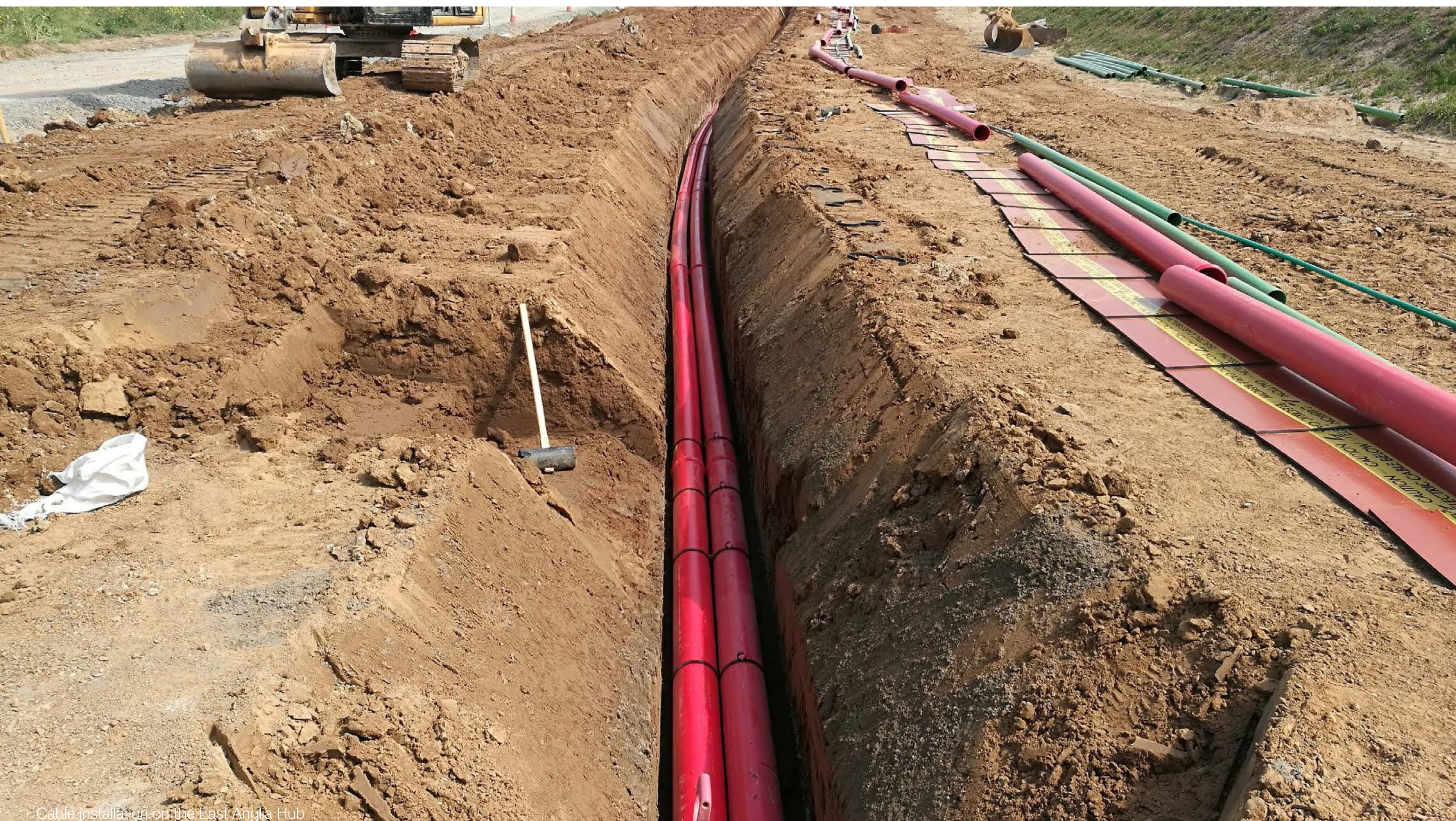
Cable installation on the East Anglia Hub
